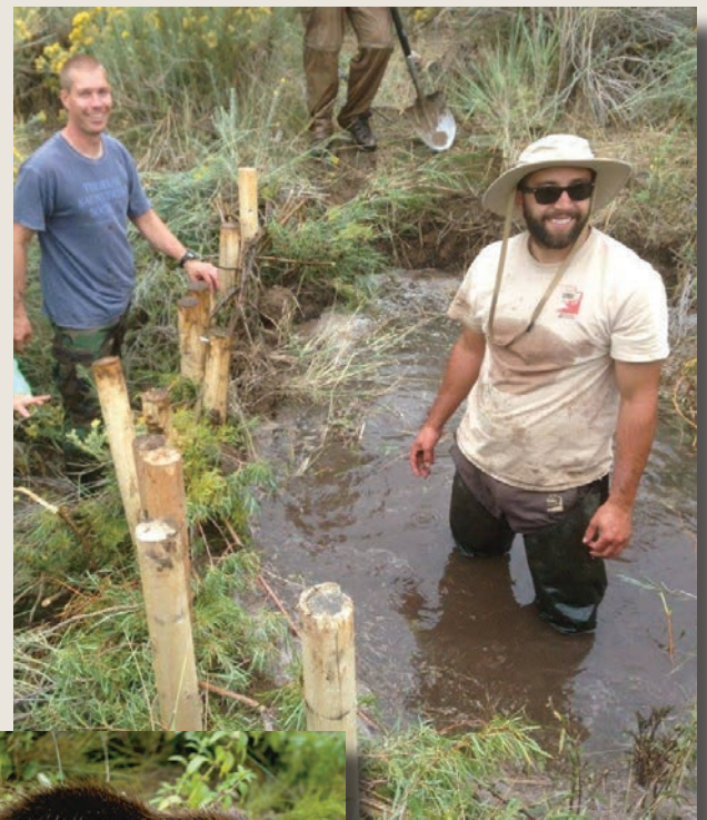
Citizen scientists create beaver dam analogues (BDAs), man-made structures that function much like beaver dams, in the Sheeprock Mountains of Utah.
